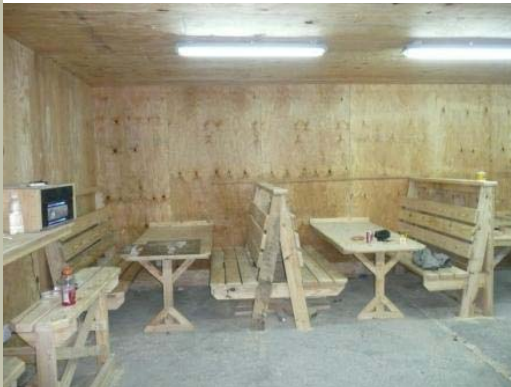
JSS Adhamiyah Dining Area After Construction
