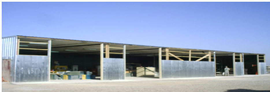
Construction Materials Yard pole barn completed
