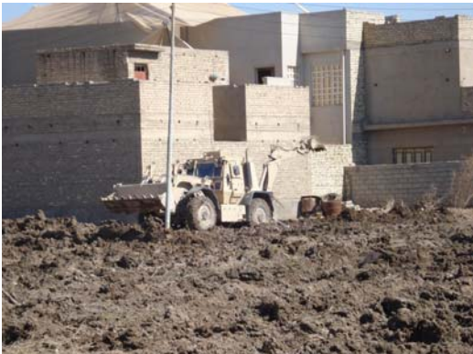
Coalition Outpost Kafayat during construction
